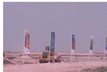
Infrastructure commences at White Bay
