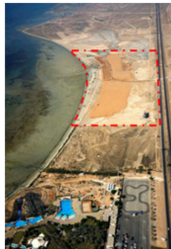
White Bay, Umm Al Quwain phase one highlighted in red with Dreamland Water Park in the foreground
